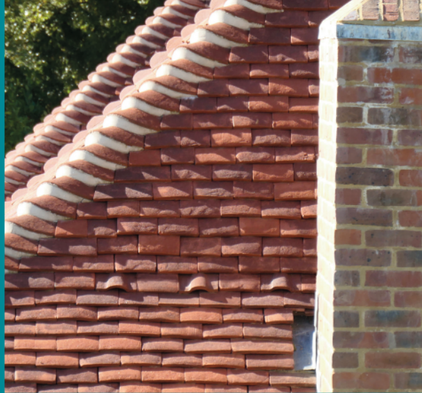
Discreetly positioned handmade clay Bat Access Tiles
